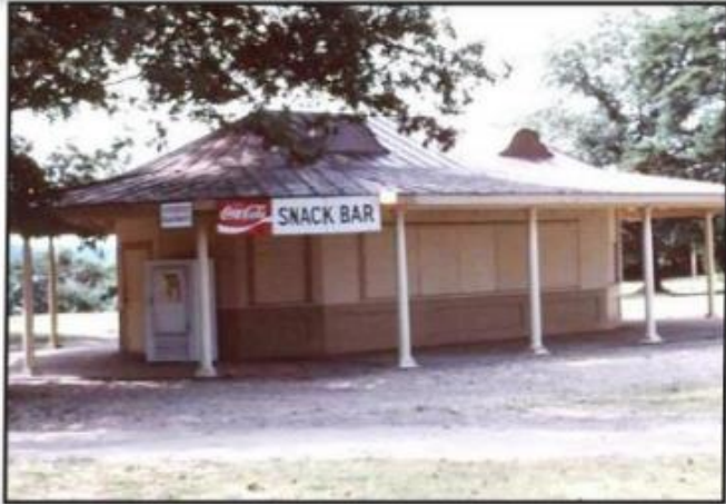
Figure 111. Picture of concession stand (AA-898D) prior to Hurricane Isabel damage taken in 1984.
