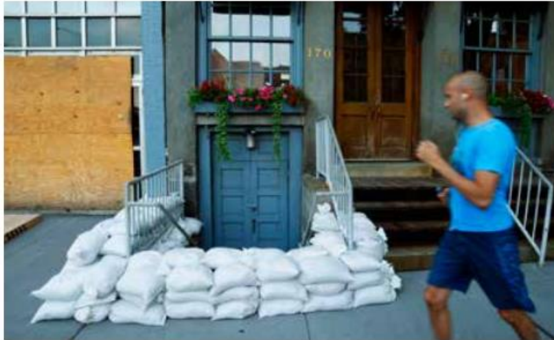
[20] Temporary measures such as sandbags can be a simple and inexpensive solution for protecting buildings in low-lying and vulnerable areas, but they are not meant to withstand moving floodwaters for extended time periods. Photo: Eduardo Munoz/Reuters
