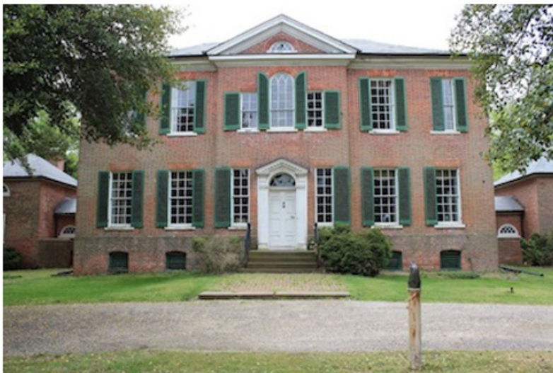
Photo 1 of 10: Front Façade, camera facing southeast.
